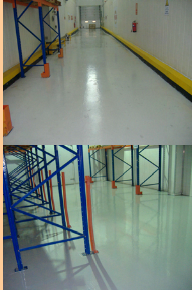
Pictures above: Refurbishment work completed
